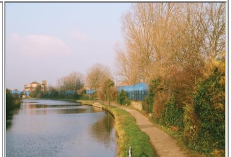
12. Hackney Cut - White Post Lane bridge in distance
